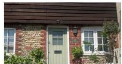
Half timber framing and half flints combined with red bricks
