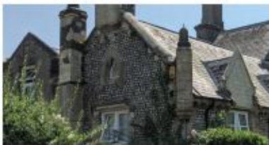
Flint work with flint chipping (galleting) to the joints
