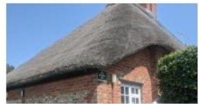
Thatched roof (made from straw)
